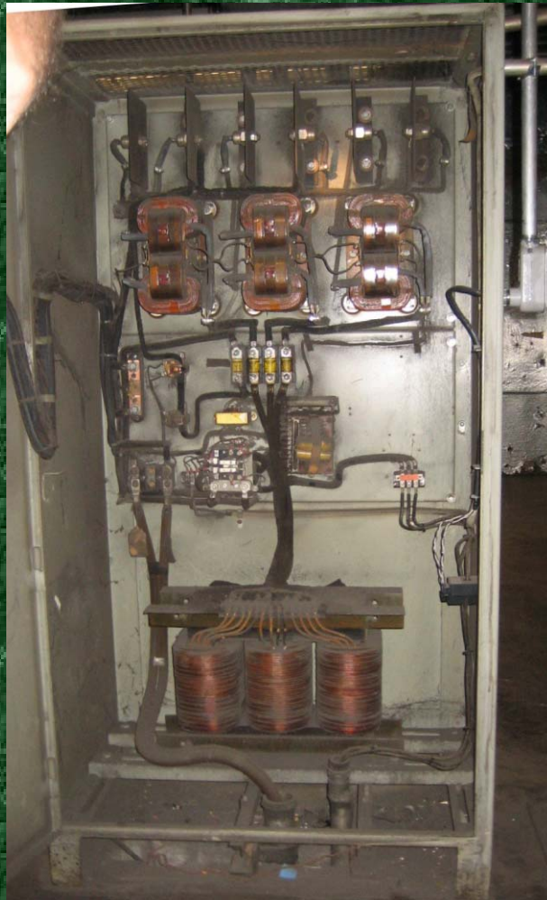
Ferroresonant Charger
